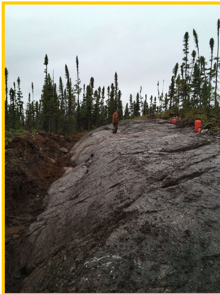
Figure 23b. Overburden stripping, GoldenEye prospect, north Sakami property, James Bay Territory.
